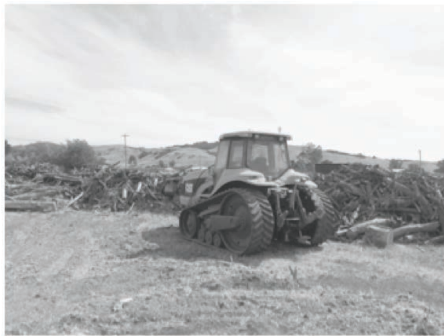
No permits needed to bulldoze trees for growing hay
